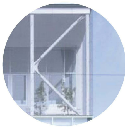
B- WHITE STEEL STRUCTURE
