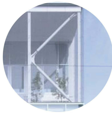
B- WHITE STEEL STRUCTURE
