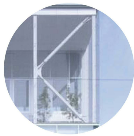
B- WHITE STEEL STRUCTURE
